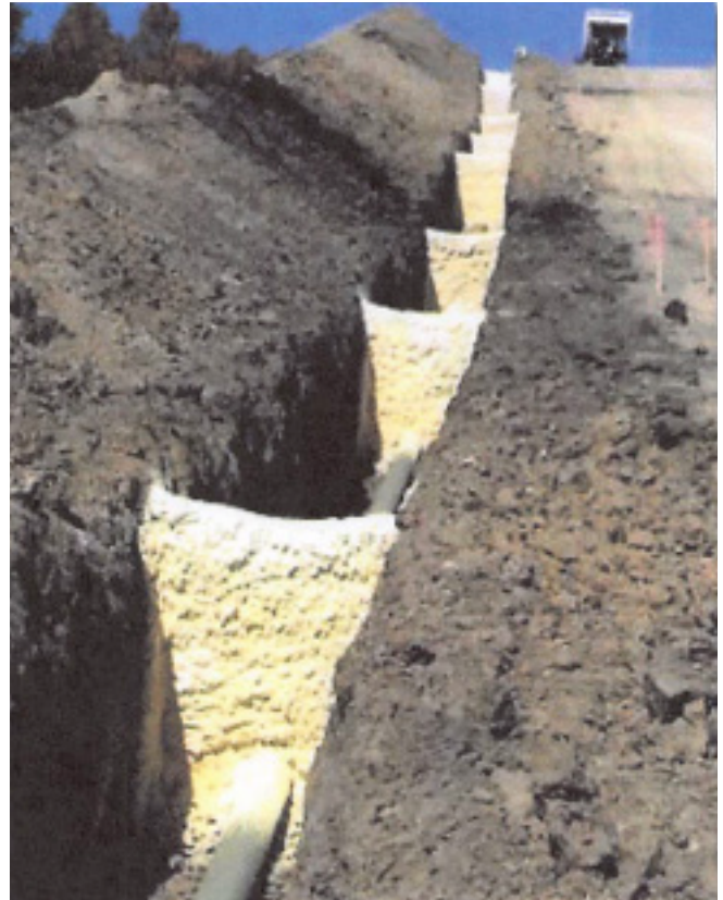
PolyLift™ trench breakers or water stops control water flow through porous soil material and improve pipeline stability.
